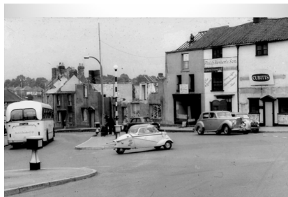
Bath Hill circa 1960 beginning of demolition
